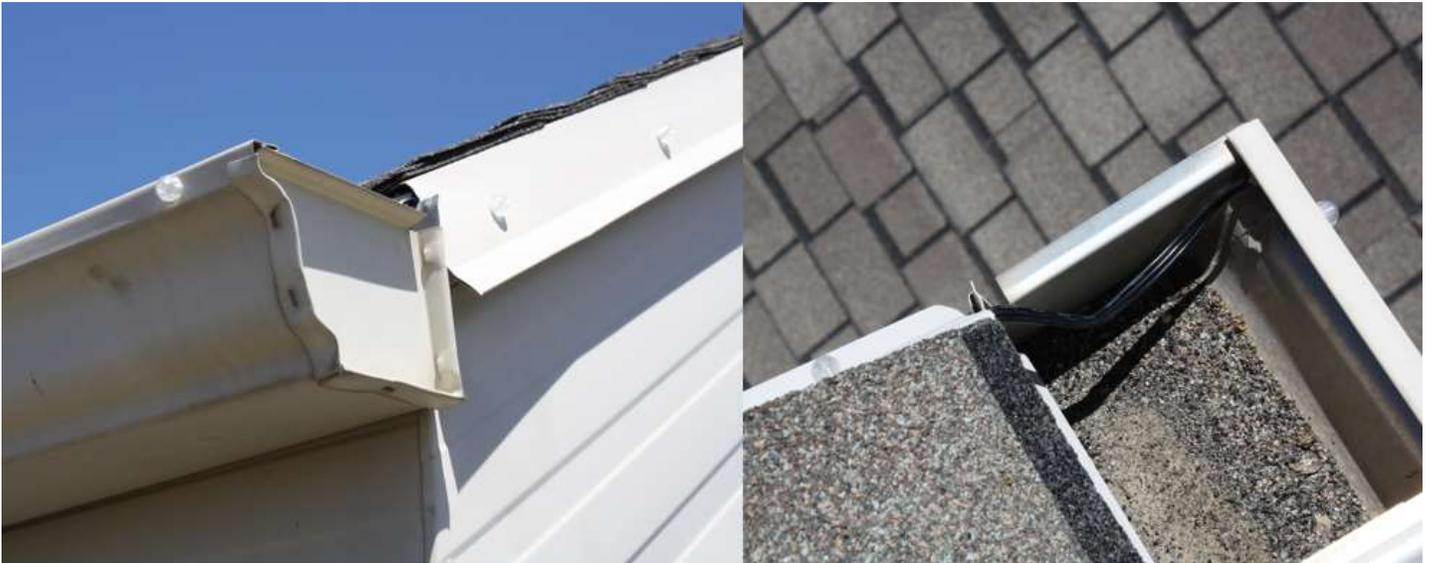
In many transitions from gutter to flashing, it is possible to install the lights without adding a small jumper section if you properly plan out the locations of the lights before drilling. While avoiding a jumper will save time with connections, be careful not to put the lights too close to the edge where the shell around the light could be exposed or get in the way.
