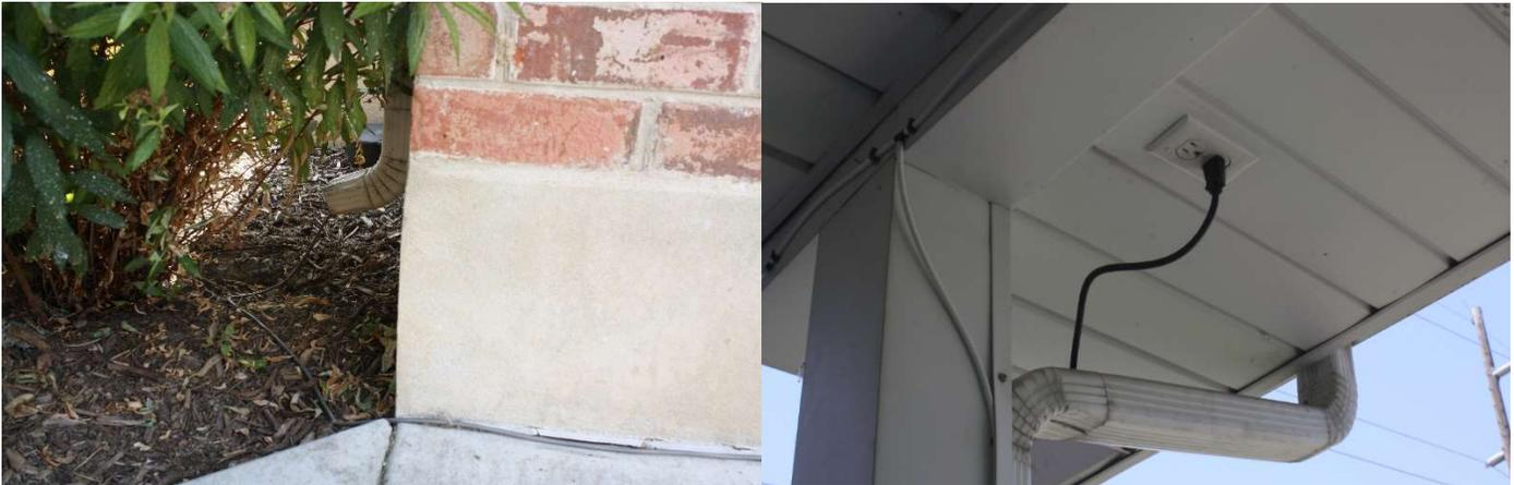
Hiding in plain sight is the mantra of EverLights. However, it's best for the power wires to hide out of sight. Running wires inside a downspout, along a siding seam, or in a dark corner are good places to hide the wires needed to span a distance.
