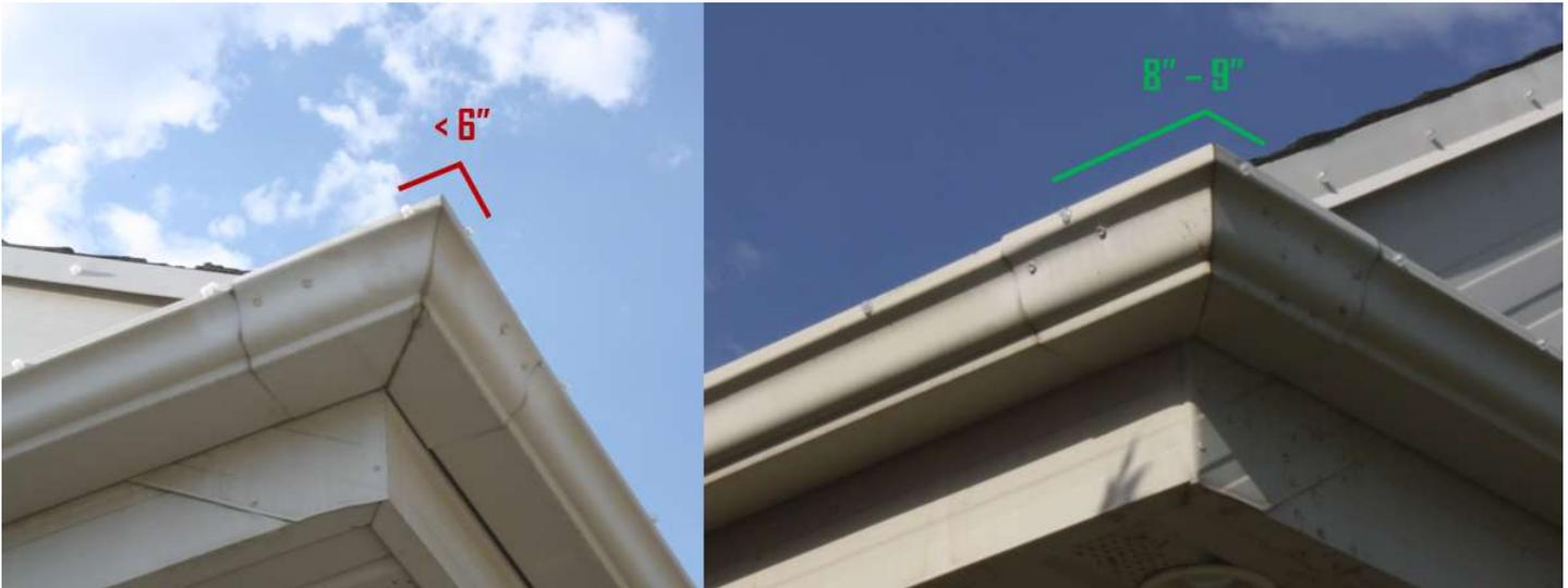
It is tempting to always start 2" from an edge so that you can put up as many lights as possible. However, the final product looks much better if you keep the consistent nine inch spacing around all corners. It's fine to cheat it down to 8" or even 7" if it helps avoid hitting gutter clips or nails, but anything 6" or less looks out of place.
