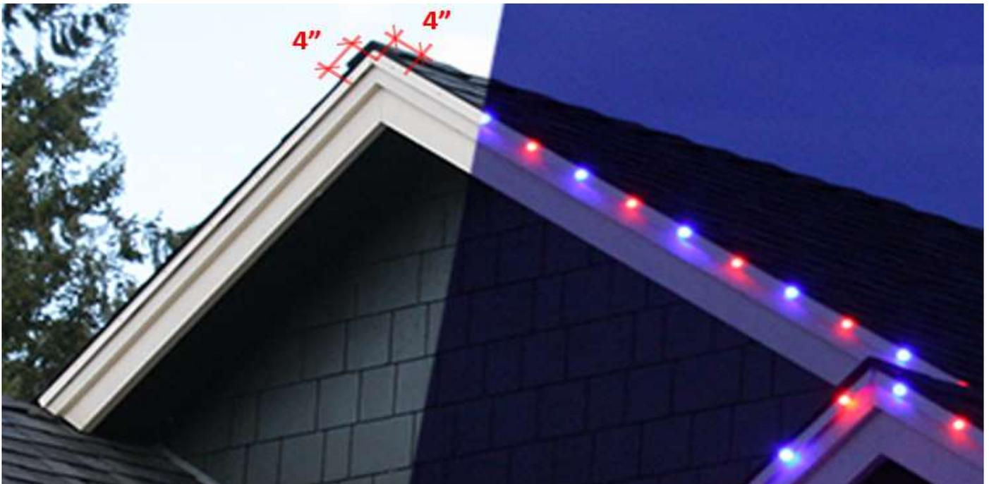
Spacing of lights at the top of eaves is critical for a quality appearance. We recommend starting the eave layout at the peaks, four inches down on each side.
